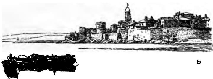
VEGLIA, SHOWING THE CASTLE TOWERS
